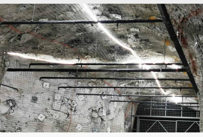
Keeping explosives underground in close proximity to operations poses a serious risk to the safety of miners. FSG Systems has developed and installed a fully functional, quick response, electronically actuated Water Deluge system for an Underground Explosives Magazine. The system is designed so that all sprinklers in the area will discharge water in the event of a confirmed fire event, resulting in complete saturation of the entire area.
