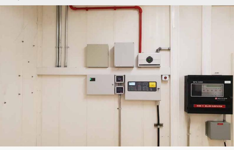
FSG Systems developed and installed an ASD Early Warning Smoke Detection System combined with a pre-engineered FM200 Gas Suppression System with electrical actuation for 12 critical electrical infrastructure rooms.
